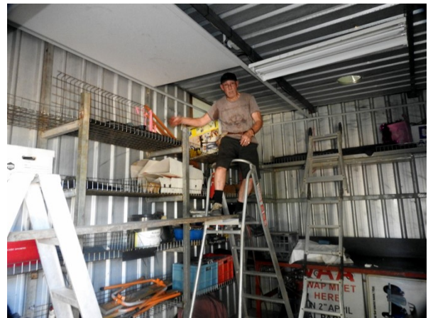
Graham installing roof insulation panels into the Engine room.
